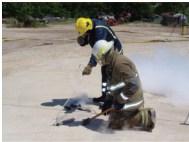
A carbon steel pipe is next taken from the LNG pit.
