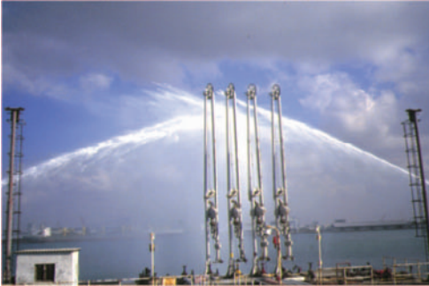
Jetty elevated monitor streams should be capable of reaching the fire hazard area (ship manifold and loading arms area under all wind conditions). This may require more than two monitors in practice. (Photo courtesy Resource Protection International)
