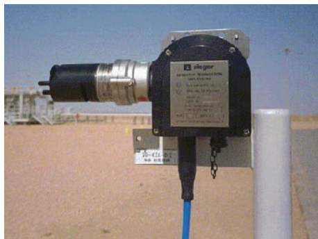
Photograph example of a point IR detector. Photo courtesy Resource Protection International.
