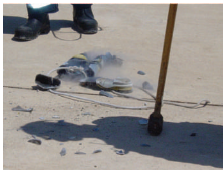
Remains of the steel pipe in the foreground.
