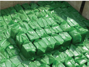
Foam glass blocks within an LNG pit. The blocks should be rested on a grid above the pit base, to allow water drainage. Picture courtesy Pittsburgh Corning
